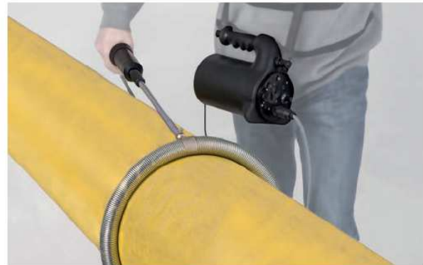
Figure 4: Application at isolated pipeline
